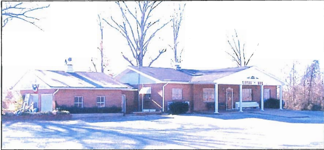
Front View of Commercial Building
