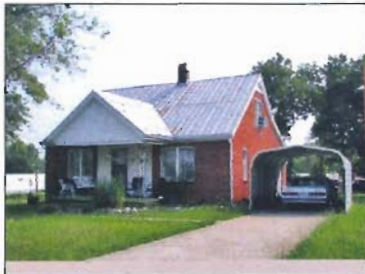
House & Portable Carport
